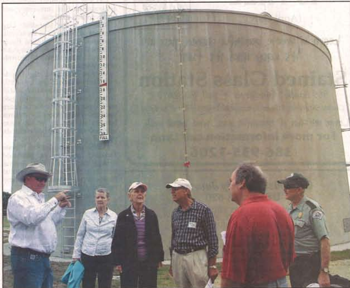
Doyle Frierson, superintendent of operations for the City of Fanning Springs, gives city residents a tour of the new centralized wastewater treatment facility on Monday.
