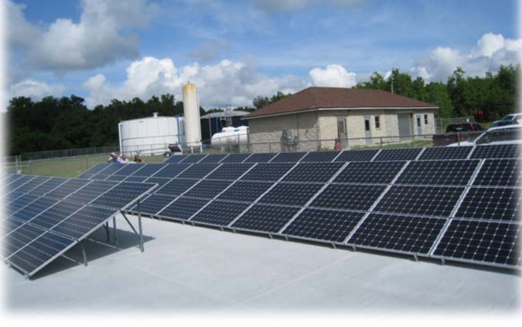
Phase I - PV collector panels with the water treatment plant in the background
